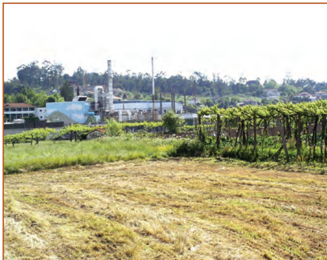
The TMG SPE industrial cogeneration plant at Vila Nova de Famalicão in Portugal feeds electrical power to the grid and generates process steam for the adjacent textile works.
