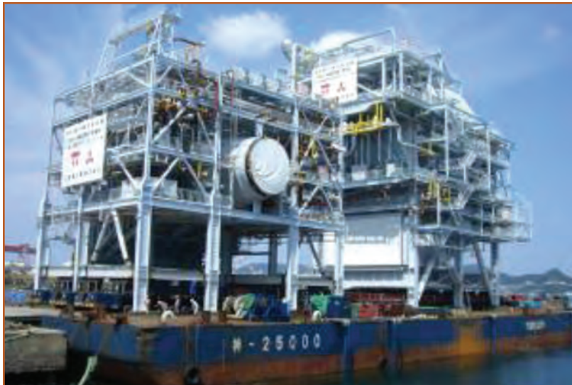
The 3800 ton HRSGs were designed and built with a modular approach to reduce assembly at site; they're shown here being moved by barge from the MHI shipyard in Nagasaki, Japan.
