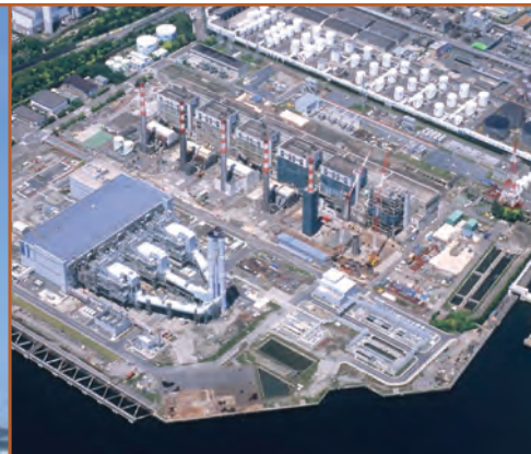
Aerial view of the TEPCO Kawasaki Combined Cycle Thermal Power Station.
